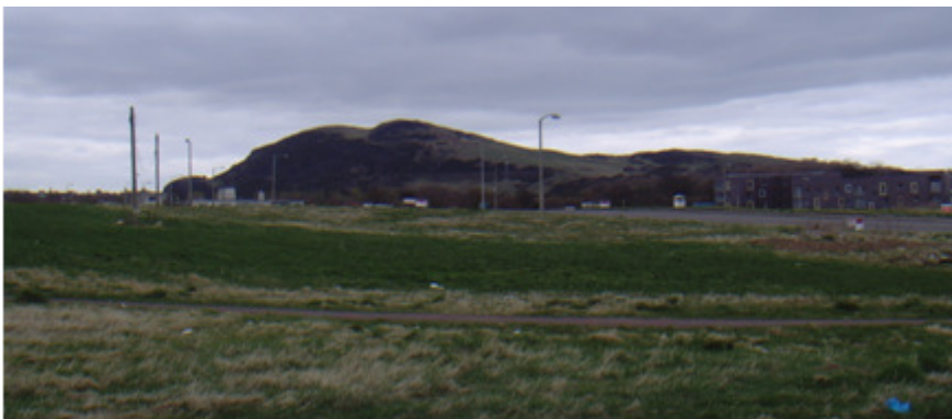
Figure 6.26 EdinburghB - Part of Area X after complete demolition (Photo by Author: March 2011)
